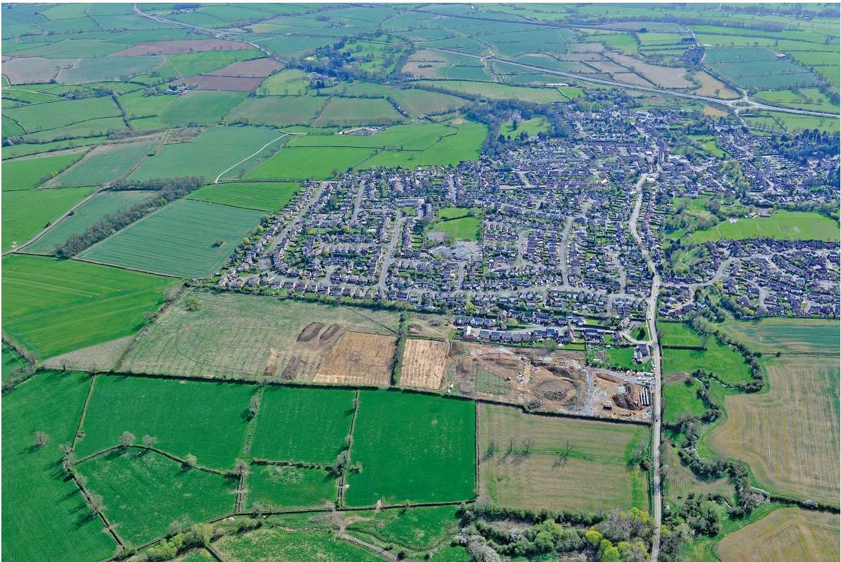
Plate 1: Aerial view of the wider setting of the development area
