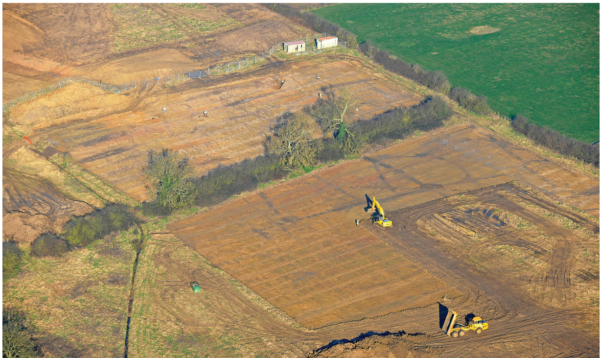
Plate 3: Aerial view of excavation area
